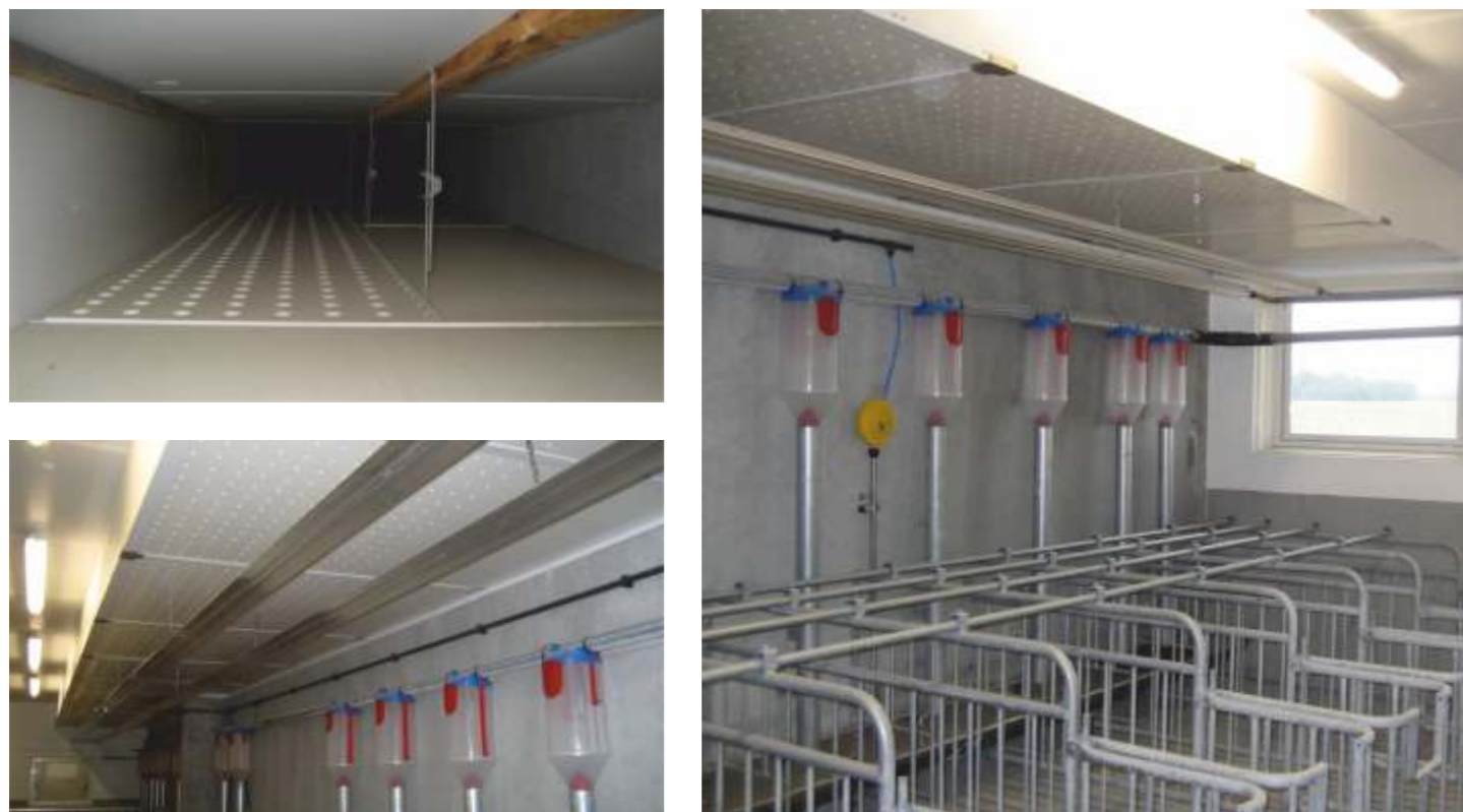
Fresh air supply via suspended perforated ceiling
