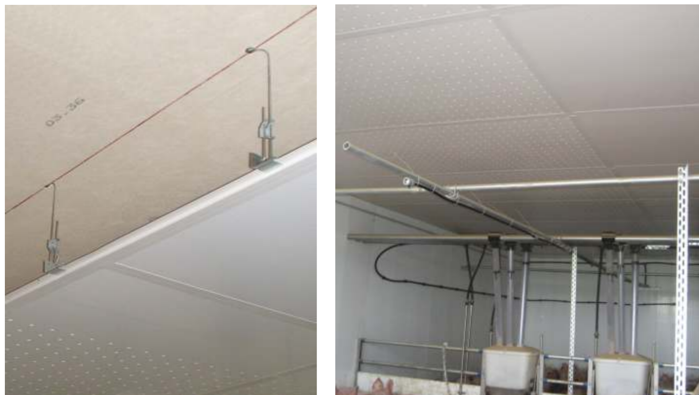
Fresh air supply via suspended perforated ceiling
