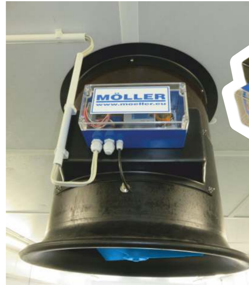
Pipe fan with damper flap
