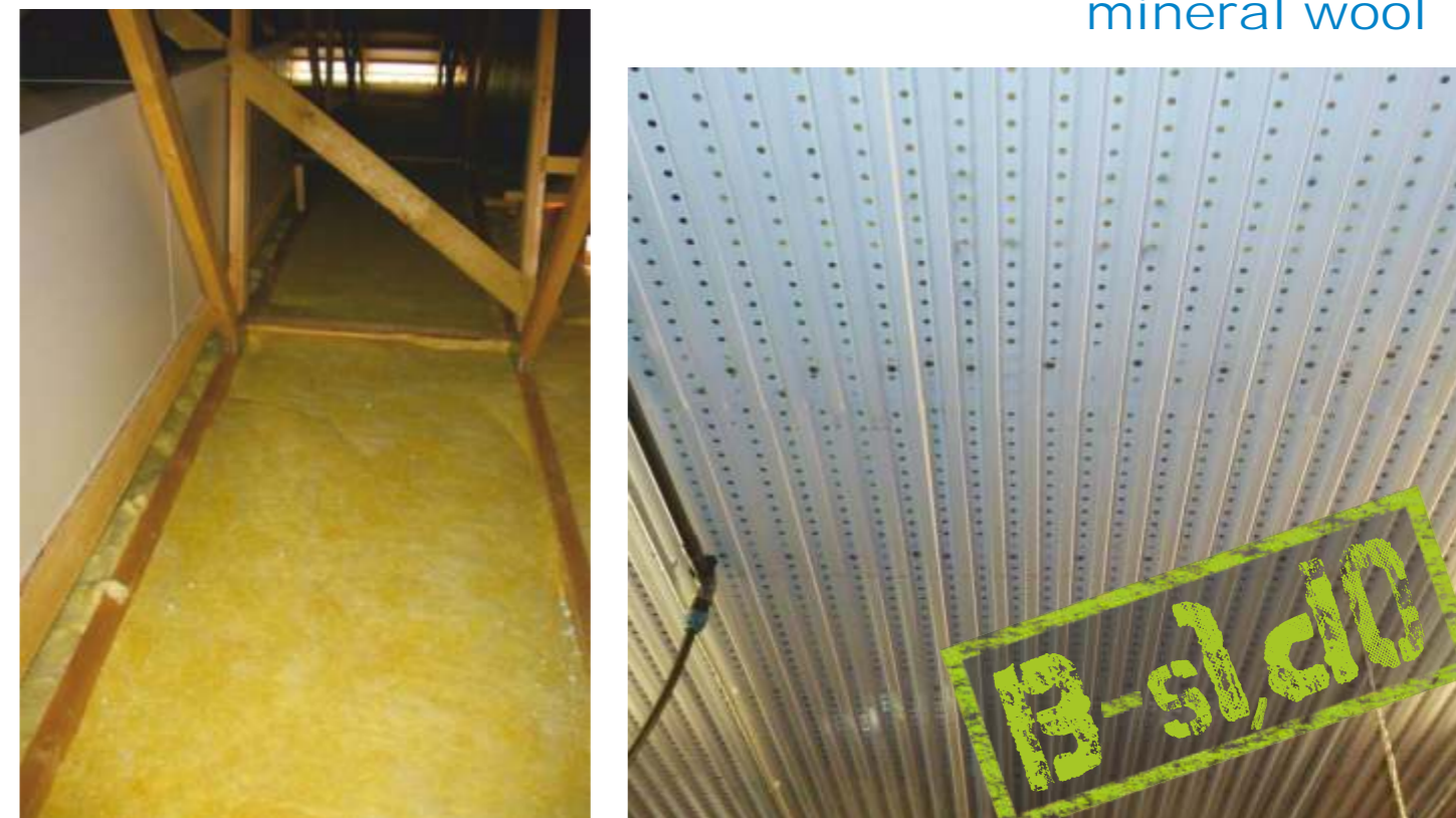
Fresh air supply via perforated trapezium ceiling with mineral wool
