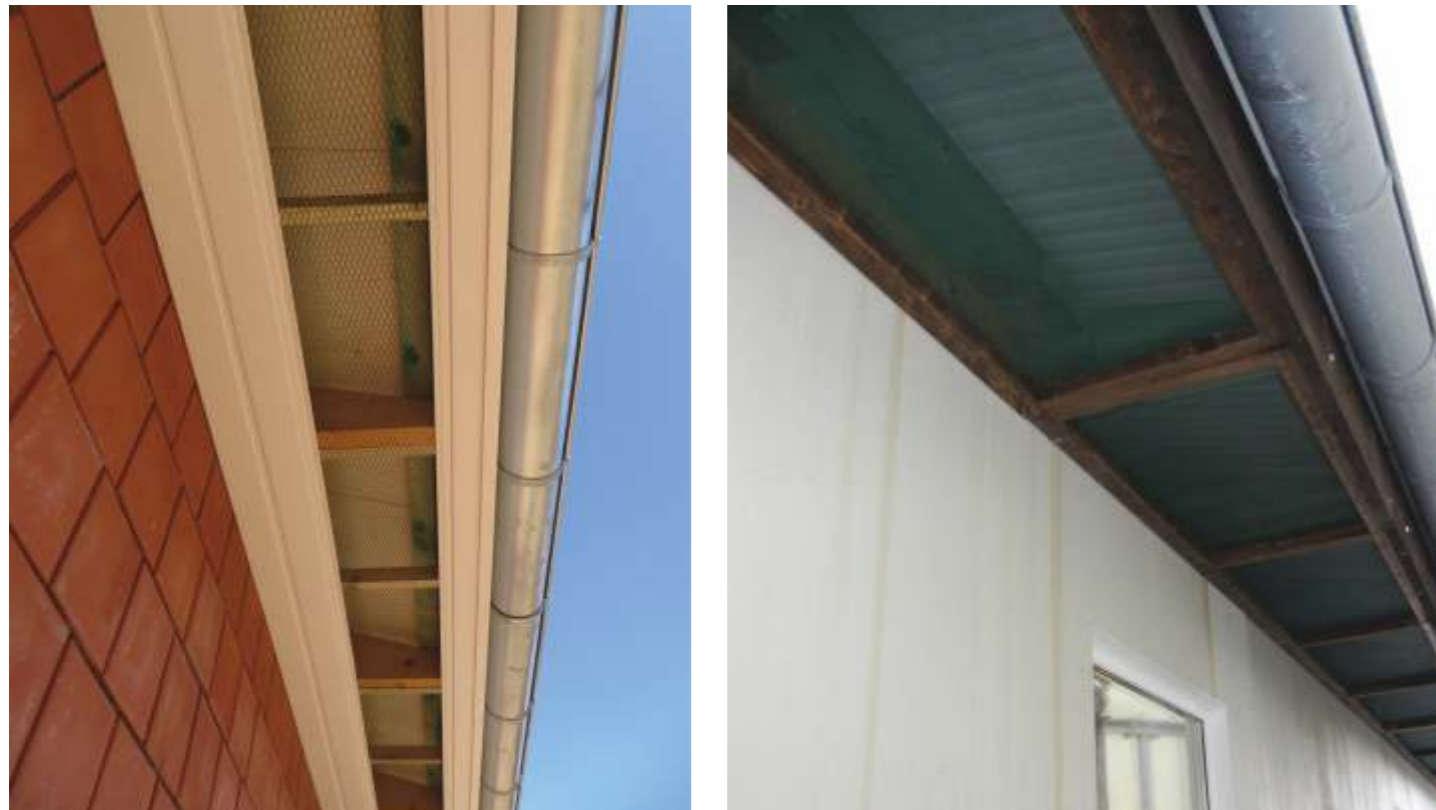
Fresh air supply entry via insulated attic
